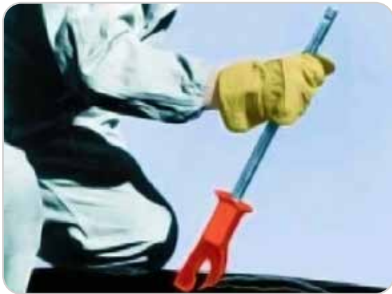
3. Loosen rubber insert with chisel.
