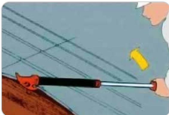
7. Breaking up roof, sheet metal.
